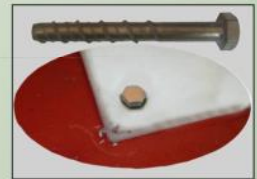
Anchor bolt in Sloping Musoir
